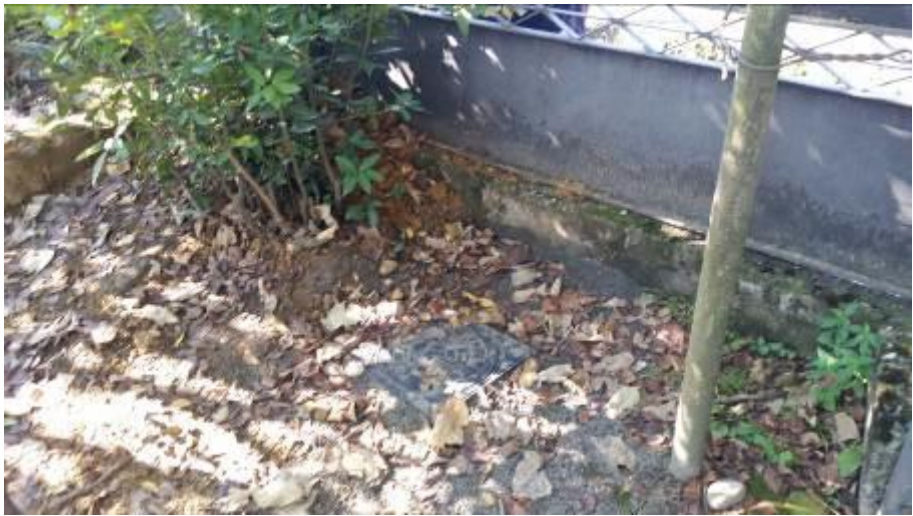
New manholes in the street of Zugdidi and private yards
