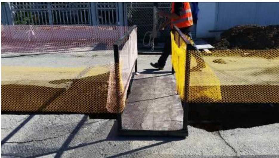
Rehabilitation of Sewerage Network in Asatiani street in Zugdidi
