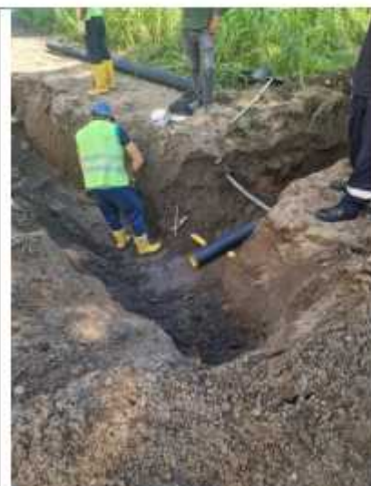
Worker without helmet and person without PPE at the construction site
